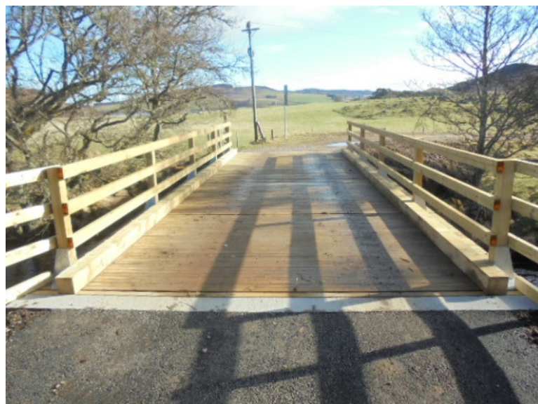
Bridge deck formed using stress laminated timber panels
