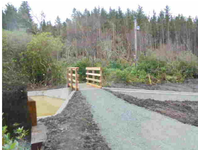
Footbridge over spillway
