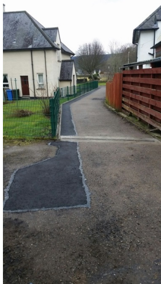
New aco channel and kerbing to address drainage problems
