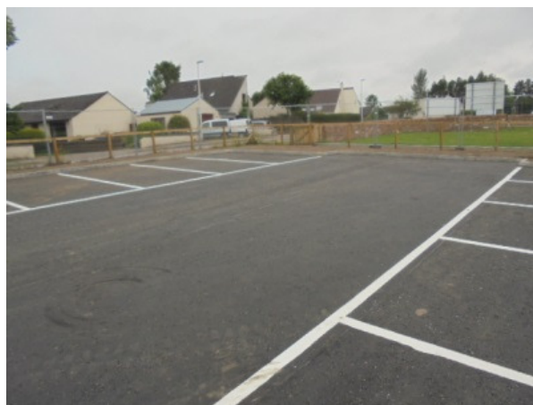
Car park extension to Craighill Primary School
